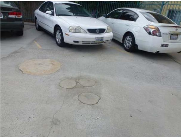
27. Reported boreholes from seismic tests conducted in subject property parking lot.
